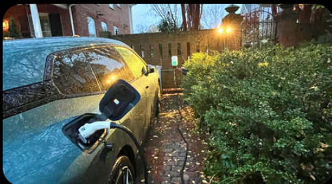
EV Charging Station
